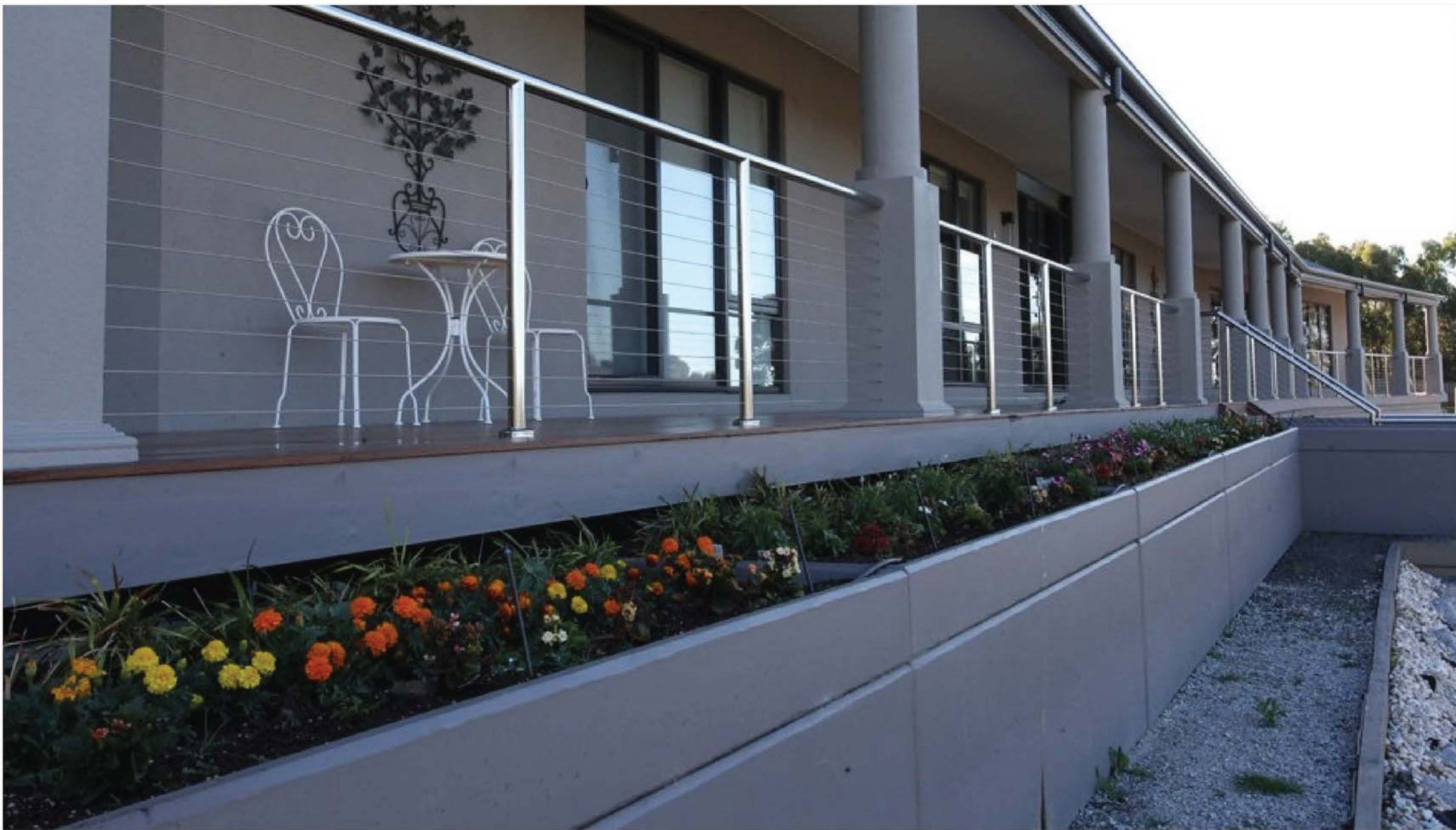
Retaining wall, garden bed and water storage. Placed hard against the house veranda and in doing so, cleverly concealing foundation works
